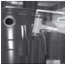
4 Attach the removed bracket to the wall and slide the unit onto the bracket.
